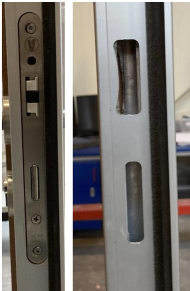
Detailed views of lock in active leaf (left) and strike plate in inactive leaf (right)
