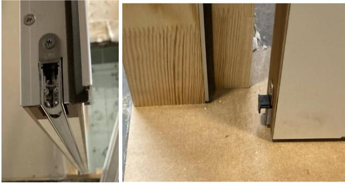
Detailed views of drop down seal (left) and actuation (right)
