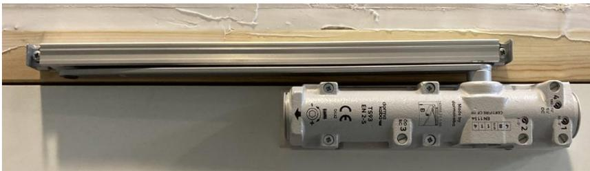
Detailed view of door closer with sliding rail
