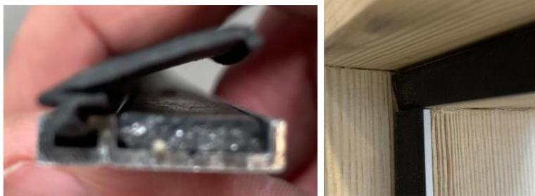
Detailed views of frame seal cross section (left) and mounting position (right)
