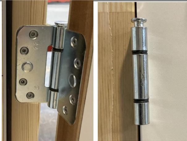
Detailed views of hinge in opened (left) and closed position (right)
